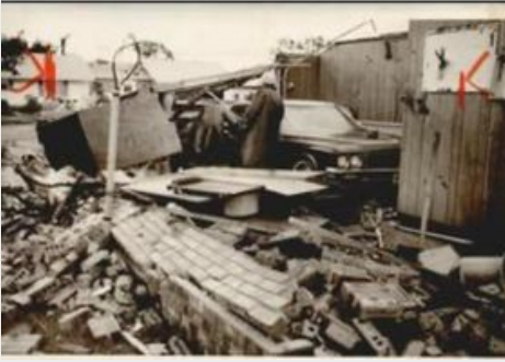
Haskell Golden checking the damage done to his home on Maple Street by the June 1974 tornado.
